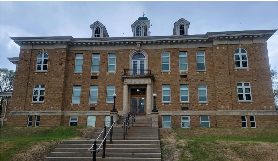
Newly Installed Metal Clad Windows and 2 nd Floor Balcony Storm Door
