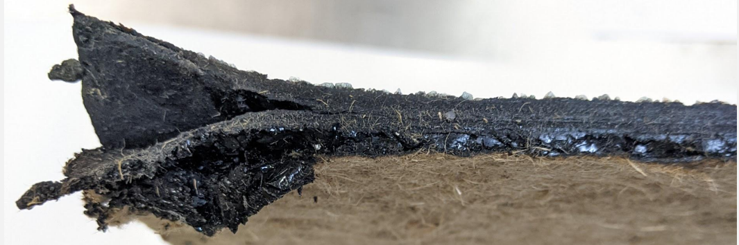
Figure 15: Municipal Services Centre West side profile.
