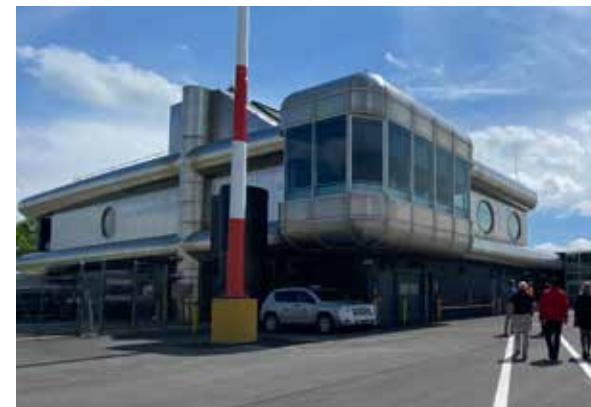
(Above) Integrated flight services facilities on the 2nd floor.
