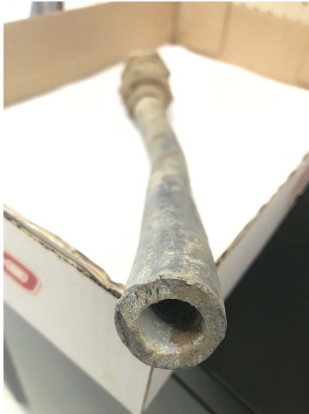
LEAD SERVICE CONNECTION CIRCA 1906 REPLACED 2011
