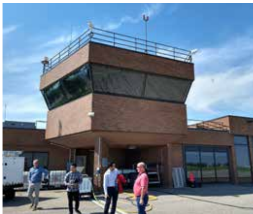
(Above) Integrated flight services facilities on the 2nd floor.
