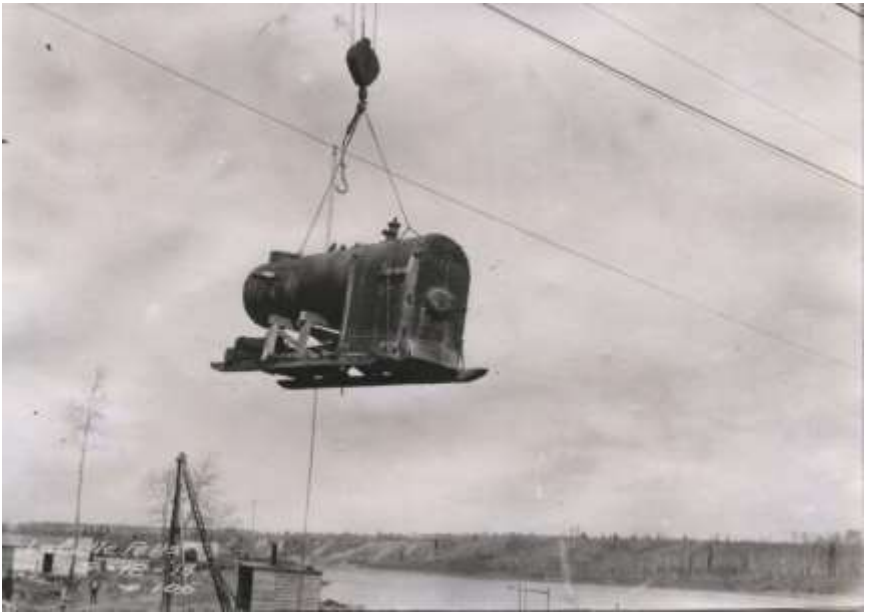
Hauling heavy materials across the river.
