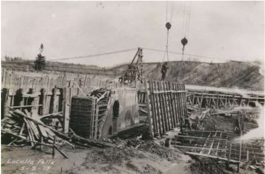
The dam begins to take shape.
