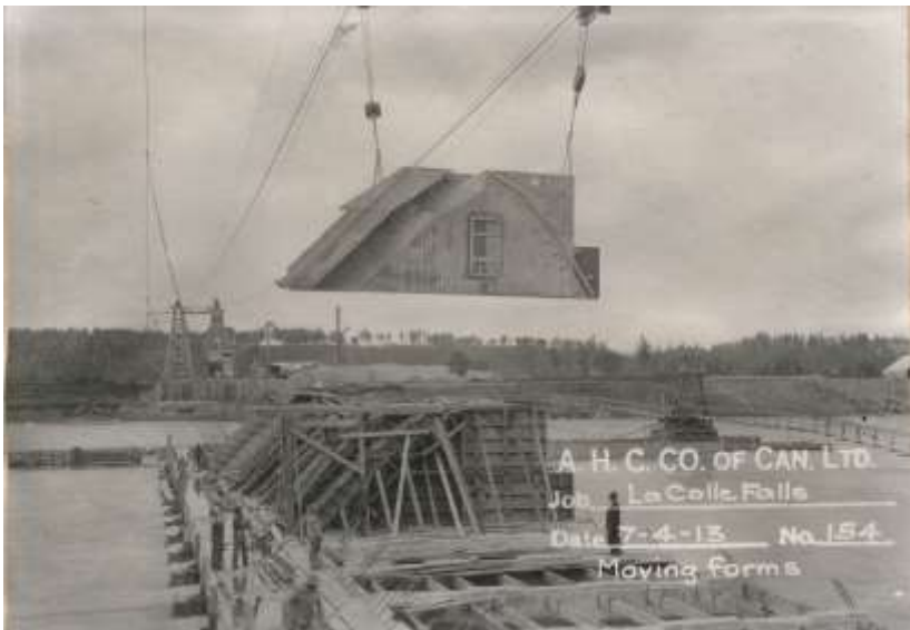
The towers and cables for heavy lifting.
