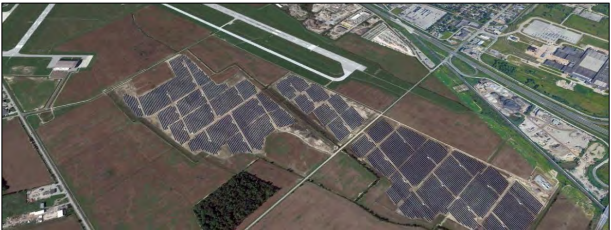
Photovoltaic generation facility at Windsor Airport (Google Earth)
