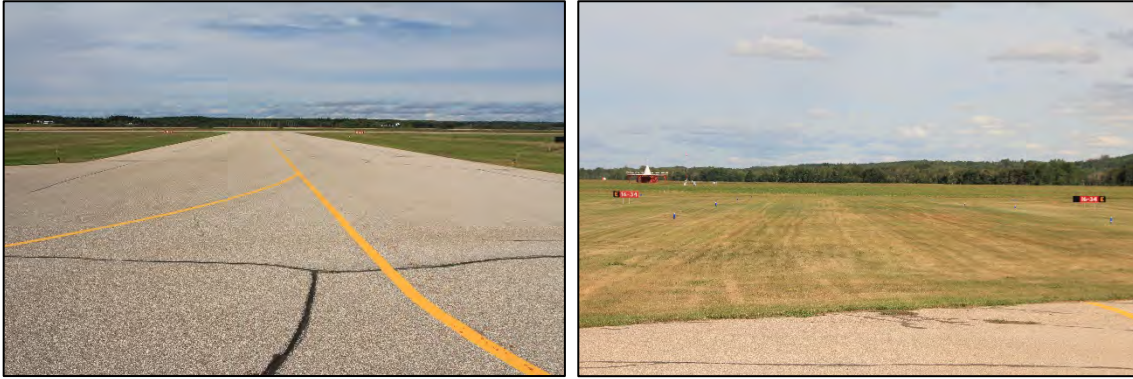
Taxiway D (left) and Taxiway E (right)
