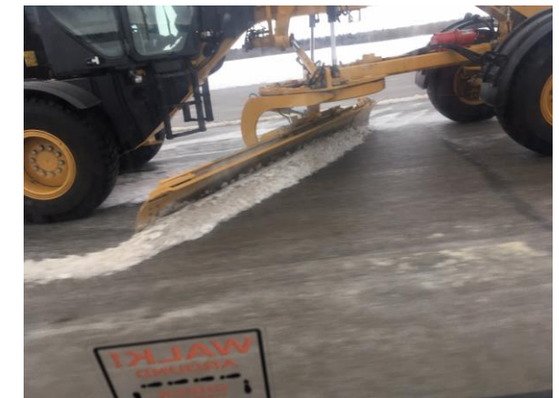
2019 Grader – Runway 1/4" of ice removal
