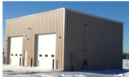
2017 Sand Shed Stores De-icing Products
