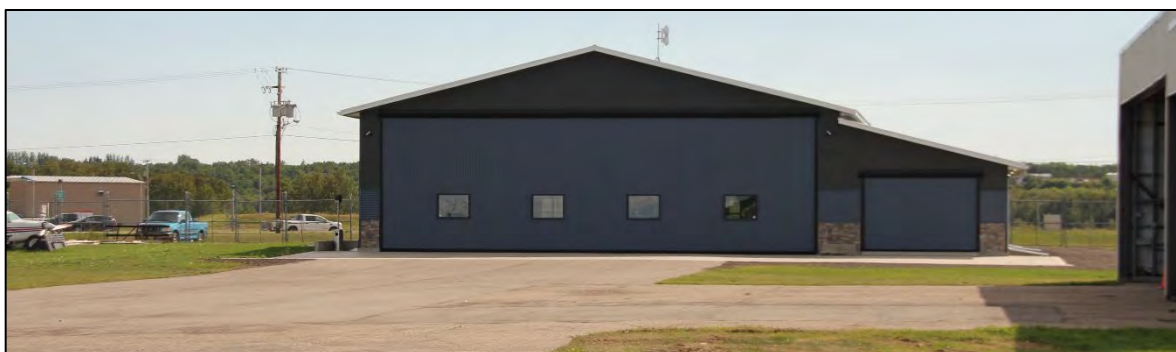
Existing airside hangar
